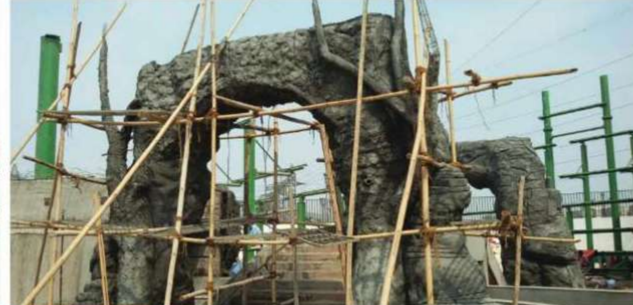
ON SITE CONSTRUCTION
