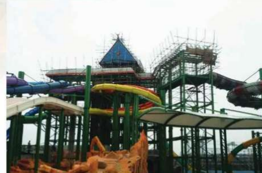
ON SITE CONSTRUCTION
