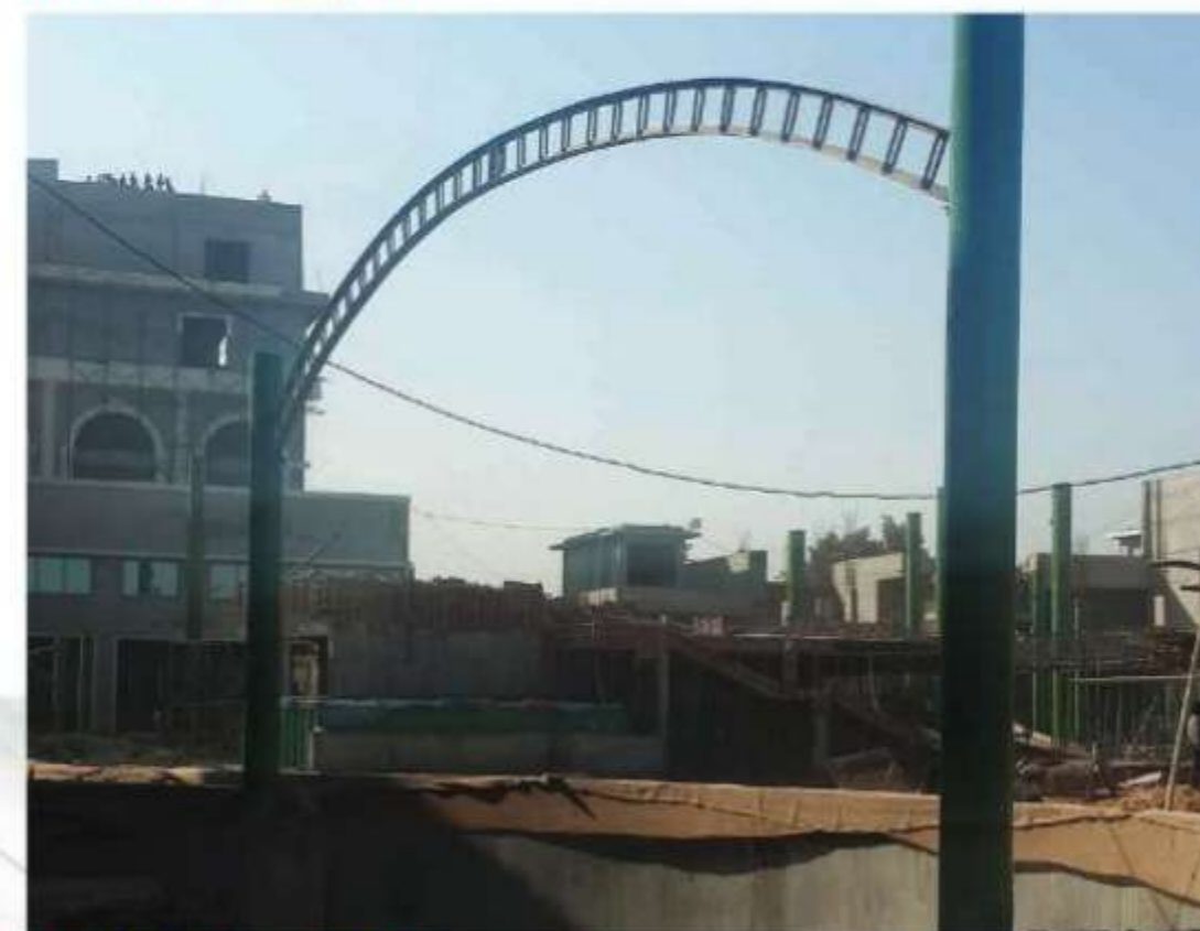
ON SITE CONSTRUCTION
