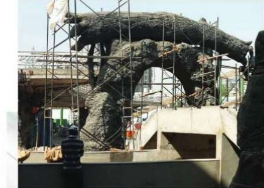
ON SITE CONSTRUCTION
