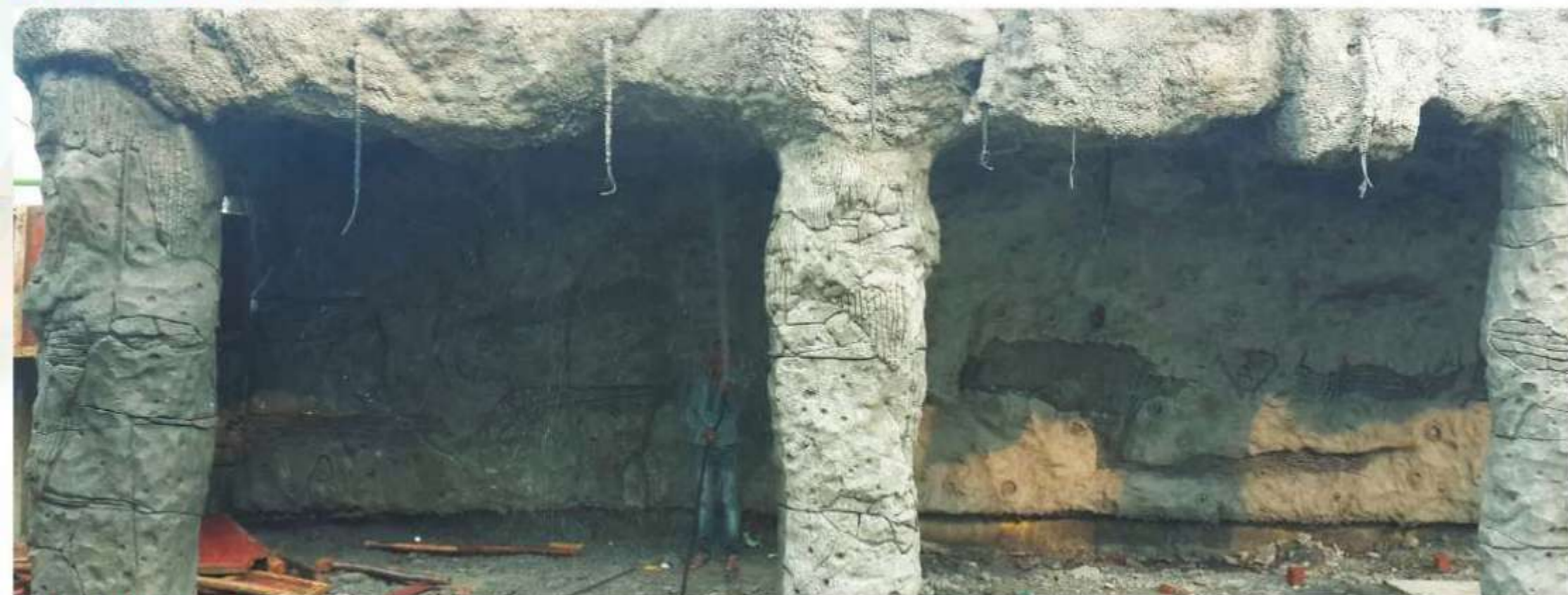
ON SITE CONSTRUCTION
