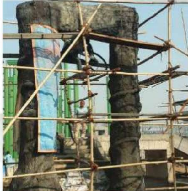
ON SITE CONSTRUCTION
