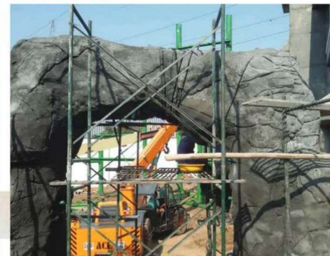
ON SITE CONSTRUCTION
